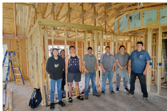
Carpentry students in the house they built.
